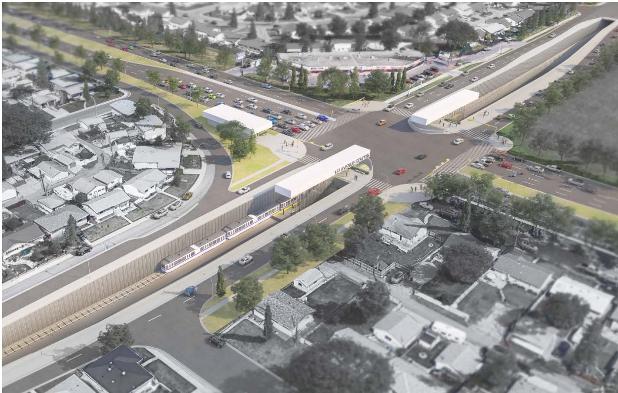
Figure 5 - Trenched Grade Separation
